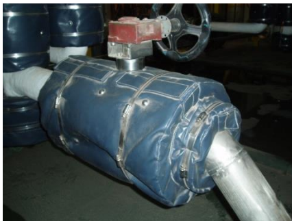
J60 Ball valve jacket on Arthit Platform
